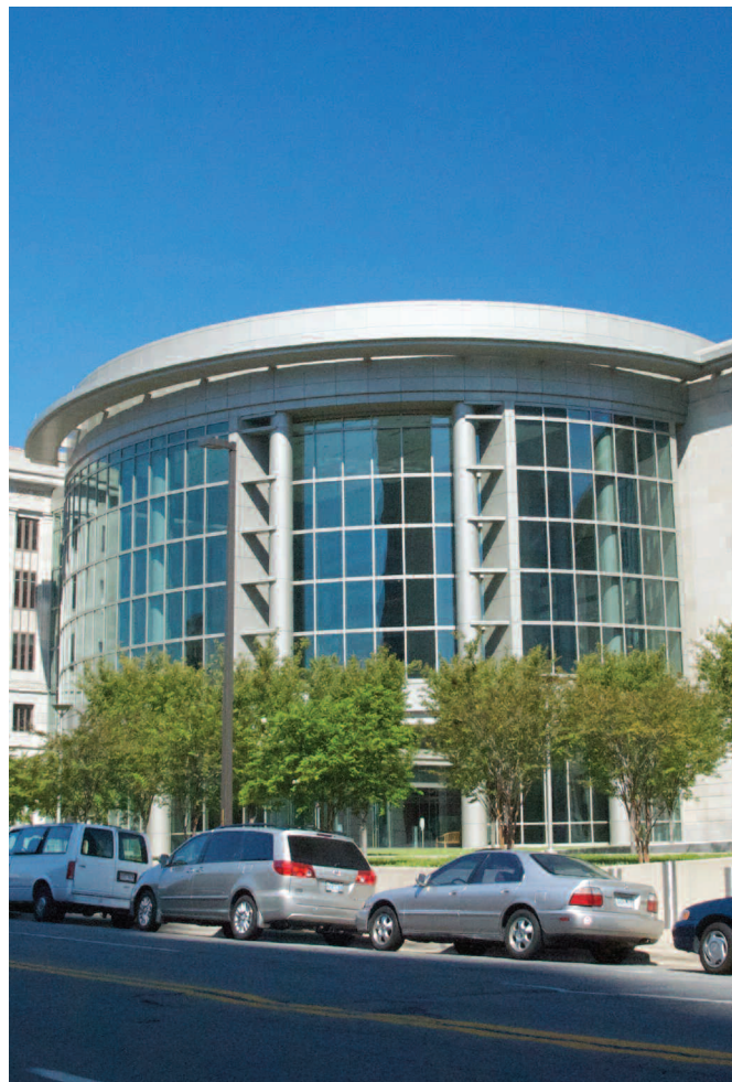
Richard Sheppard Arnold Federal Courthouse in Little Rock
